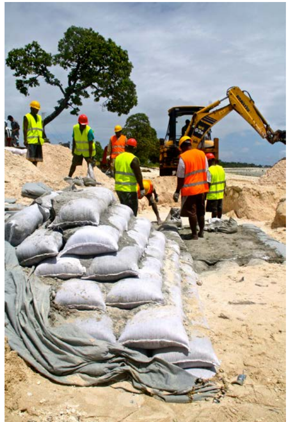
Budowa wałów, fot. Carlo Iacovino, Global Environment Facility, CC BY-NC_SA 2.0
